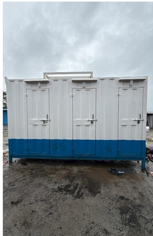
SANITARY FACILITY PROVIDED FOR WORKERS
